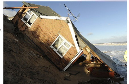
This is a house falling into the sea due to erosion.
